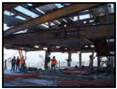
Structural Steel Erection
